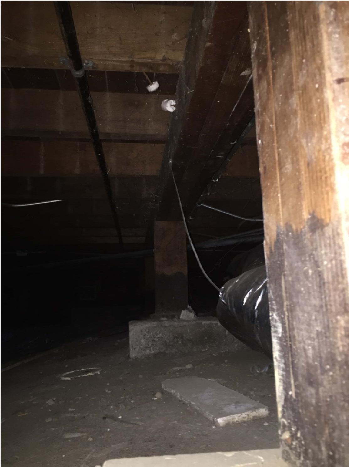
Figure 8: First Floor Framing from Crawlspace
