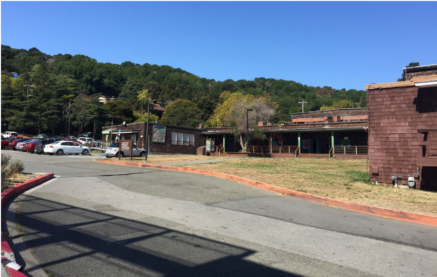
Figure 4: Existing Main Building – Manzanita Recreation Center
