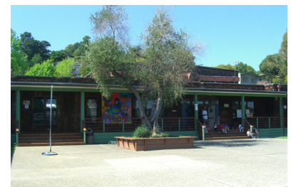
Existing Manzanita Recreation Center
